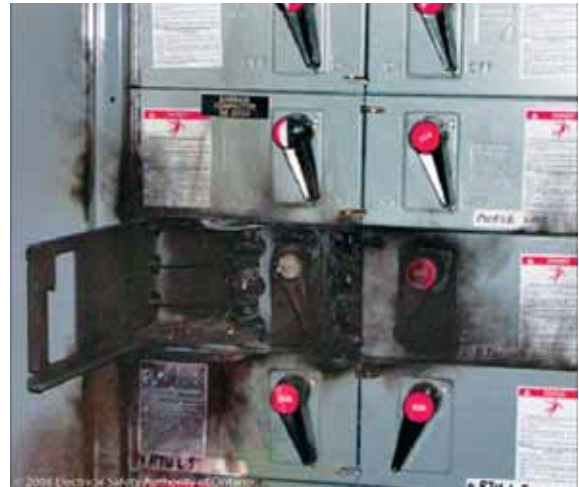
Photo: Electrical Safety Authority of Ontario
